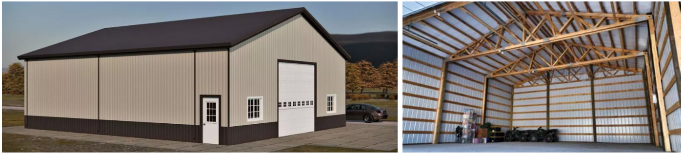
Interior and exterior example images of poles barns.
